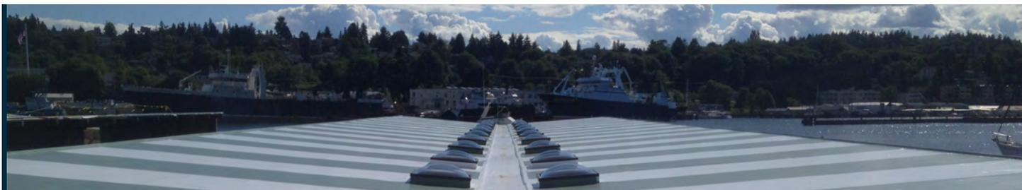
According to manufacturer’s representative Ian Murphy of Exterior Allied Systems LLC in Portland, Ore., there were several advantages to using the Fibertite RhinoBond system. “FiberTite weighs less than a metal roof and with its hot-air welded seams has better watertight integrity,” he said. “the RhinoBond system allows the membrane to be attached directly into the wood purlins under the metal panels and was an excellent way to meet the FM 1-90 wind uplift requirement.”
