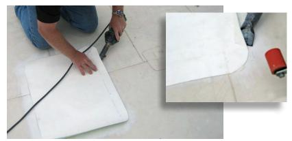
8. Weld the perimeter of the patch, ensuring a minimum 1.5" continuous weld.
