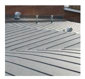
1. Plan layout of the fleece back to coincide with the layout of the SMR-Profiles.
