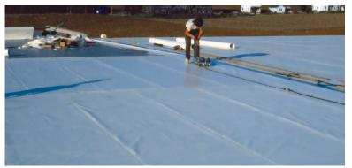
Once the membrane and the building go through a few cycles of expansion and contraction through the heating and cooling with the seasons, the fabric will relax and take on a flatter and tighter appearance.
