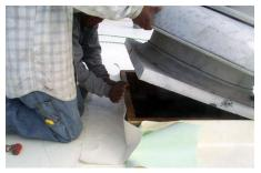
Install all four sides and weld all overlaps and the base of the flashing membrane.
