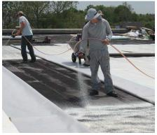
The proper technique is to slightly arc the adhesive as it disperses from the application nozzle allowing to land and spatter on the substrate.
