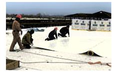
Pull the tab down snug and install fasteners and stress plates per the project specifications.
