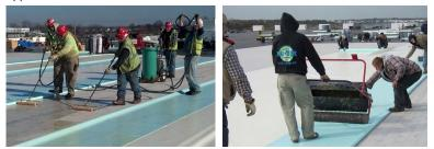
Use solvent resistant, medium nap rollers (3/8"nap) for adhesive application. Generally, 3/8" nap is suitable for both solvent and water based adhesives. All rollers shall be kept clean and free from cured adhesive.
