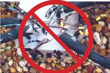
Every effort should be made to eliminate the need for pitch pans, including the removal of existing pans. Contact the FiberTite Technical Department for specific design recommendations.
