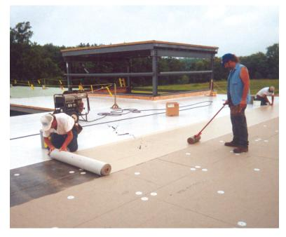
Lastly, membranes with SM style back coats (FiberTite-SM and FiberTite-XTreme) can be applied using FTR 490 in a one side, substrate only, application. The adhesive is applied to the substrate and the membrane is rolled into the wet adhesive.
