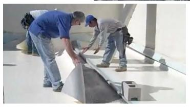
Open time for the adhesive will vary depending on the temperature and is a maximum 10-minutes but best practice is to embed the fleece back membrane as soon as possible following the application of the foam.
