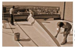
Fold the portion "making up the bottom" of the overlap into the adhesive first.
