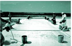
Use a weighted roller to finish mating the membrane to the substrate.
