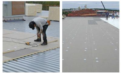
Install no more insulation than can be covered with completed (secured and sealed) FiberTite Roofing System during the same work day.
