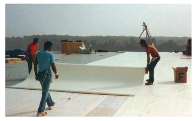
When the first 5 tabs are attached, pick up the remaining core of material and align it behind the first tab that was attached ( $5^{th}$  tab in).
