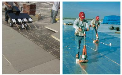
Alternatively, follow project specifications and/or FiberTite Guide Specifications for adhesive coverage and application rates when adhering roof insulation and/or cover board. Keep track of the number of containers and or the total volume of material use daily. Divide the volume into the number of applied squares of insulation to ensure adequate amounts of adhesive are being used.
