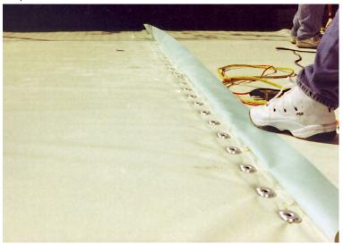
A Standard Top-Sider Roll for mechanically fastened FiberTite Roofing Systems is 20' wide  $\times$  86.7' in length for a gross yield of 1,734 ft<sup>2</sup>.
