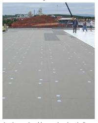
Install no more insulation than can be covered with completed (secured and sealed) FiberTite Roofing System during the same work day.
