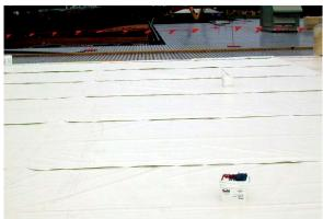
Subsequent rolls are installed with a nominal 5" overlap. Each 20' x 70.5' custom roll requires approximately 250 lf. of field welding but only 39 sf. of field overlap during installation.
