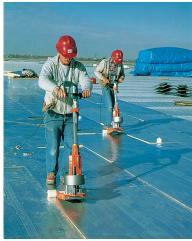
Alternatively, follow project specifications and/or FiberTite Guide Specifications for adhesive coverage and application rates when adhering roof insulation and/or cover board. Keep track of the number of containers and or the total volume of material use daily. Divide the volume into the number of applied squares of insulation to ensure adequate amounts of adhesive are being used.
