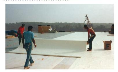
When the first 5 tabs are attached, pick up the remaining core of material and align it behind the first tab that was attached ( $5^{th}$  tab in).
