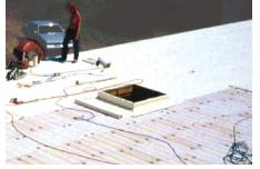
Depending on where the roll is cut, the remaining roll may no longer have any "reversed" tabs. Field reversing a tab is permitted
