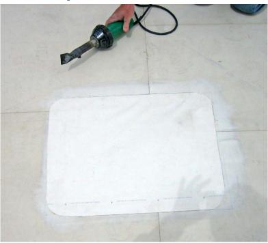
10. In the event that a field seam requires frequent or multiple patches, a minimum 4" wide strip of membrane should be welded over all the patches/the area to cover all the defects and present a more uniform and aesthetically pleasing appearance.
