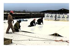
Pull the tab down snug and install fasteners and stress plates per the project specifications.
