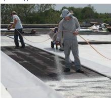
The proper technique is to slightly arc the adhesive as it disperses from the application nozzle allowing to land and spatter on the substrate.
