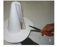
Trim off the top of the flashing, cutting along the corresponding gradient to match the pipe diameter. »
