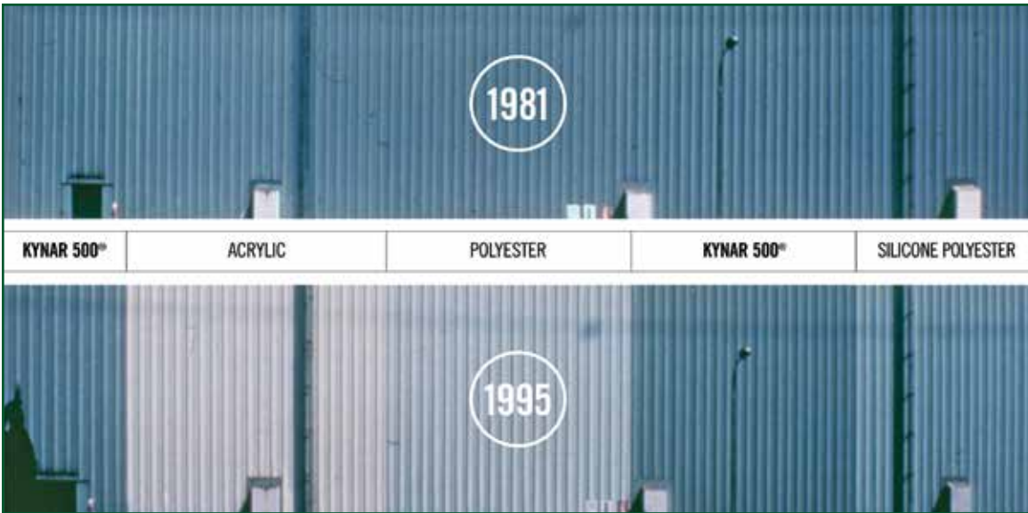
Photo 10 – Field-testing and weathering of PVDF.
