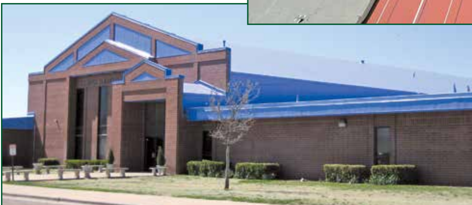
Photo 11 – Plainview Elementary School, Plainview, Texas, with its "Dazzle Blue" Kynar roofing system.
