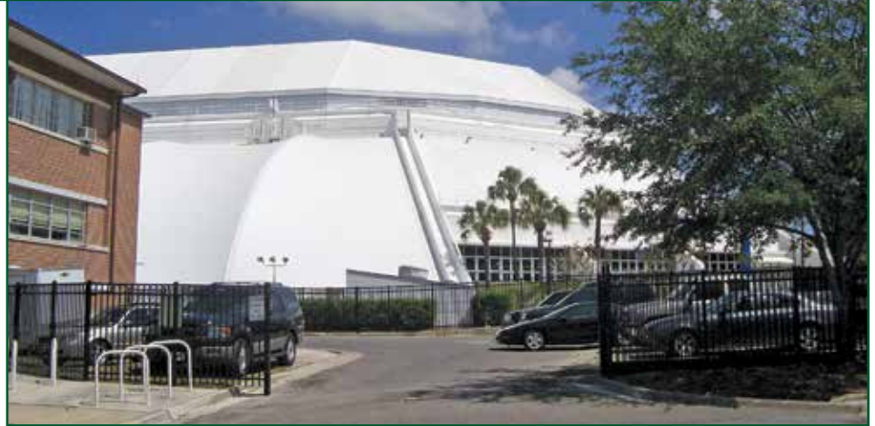
Photo 4 – University of Florida, O'Connell Center, May 2008, after cleaning. The white structure below the roof area is a Teflon-coated fiberglass.
