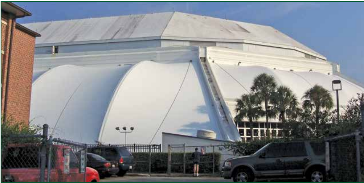
Photo 3 – University of Florida O'Connell Center, September 2005.
