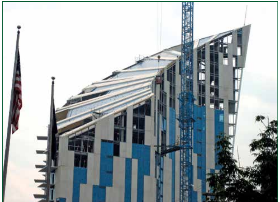
Photo 2 – The Ascent at Roebling's Bridge, Covington, Kentucky.
