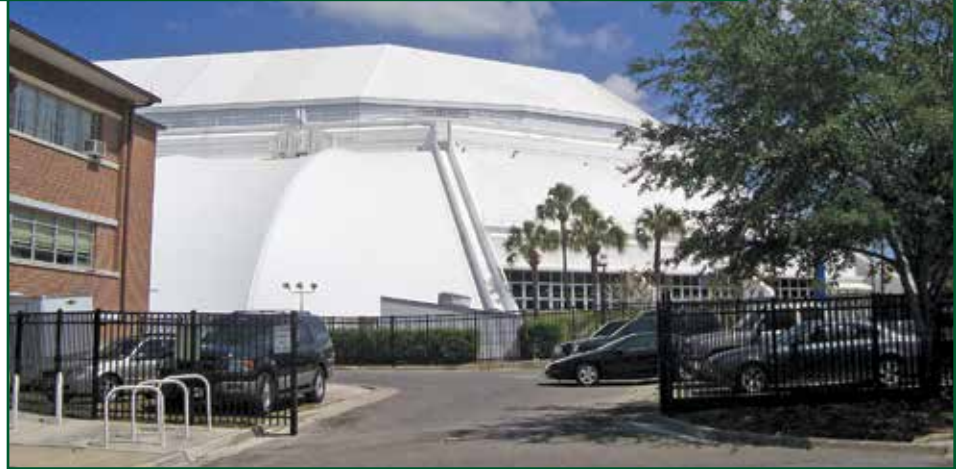
Photo 4 – University of Florida, O'Connell Center, May 2008, after cleaning. The white structure below the roof area is a Teflon-coated fiberglass.
