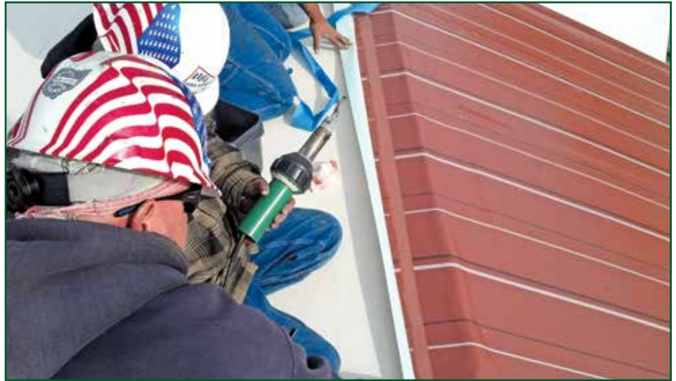
Photo 13 – Fluoropolymer removed and ready to weld.
