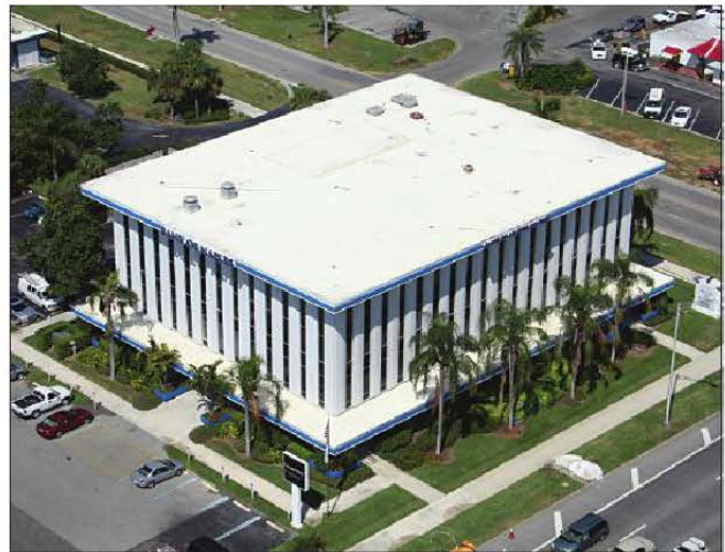
A mechanically fastened 25-year-old nominal 0.9-mm (36-mil) ketone ethylene ester (KEE) roofing system in Naples, Fla.
