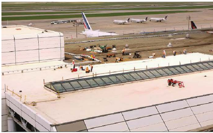
A 12,820-m 2 (138,000-sf) adhered KEE roofing assembly on an airport.
