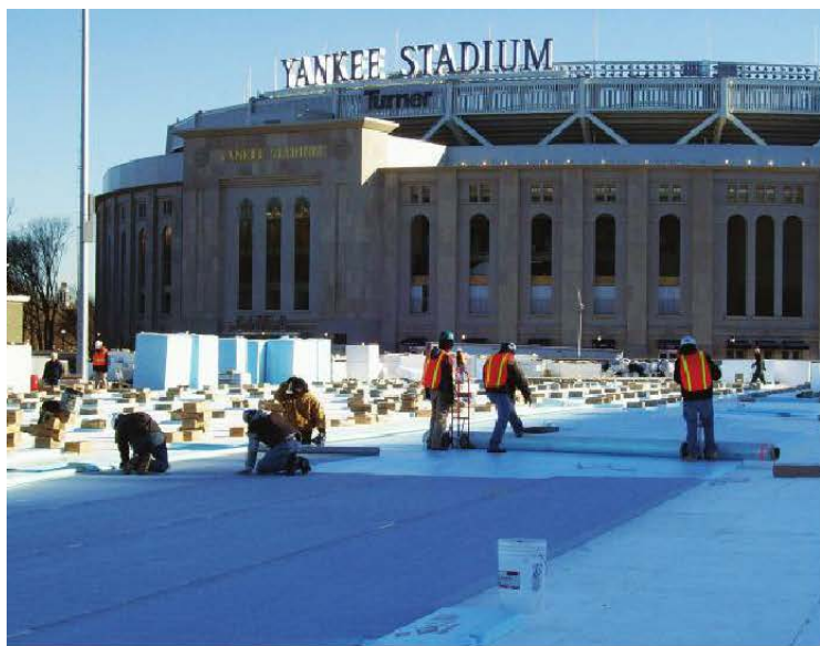
A 26,477-m 2 (285,000-sf) KEE roof installed below an artificial turf 'garden roof' at Yankee Stadium Parking Garage in New York.
