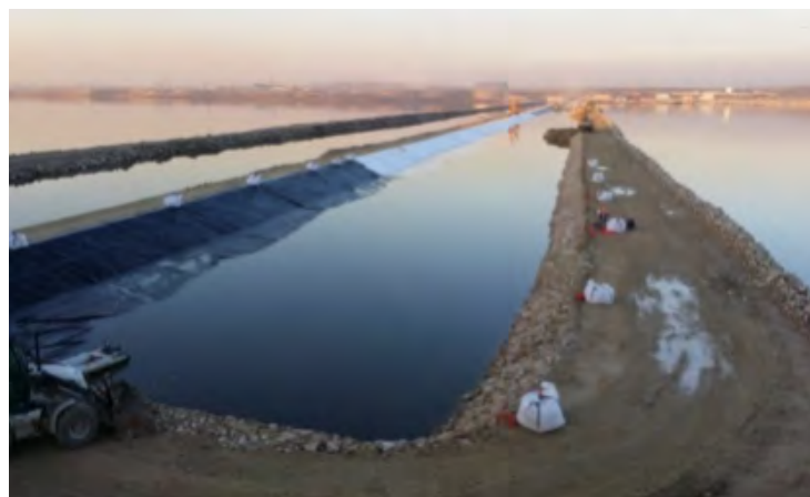
Figure 13: Road Dam Geomembrane Installation
