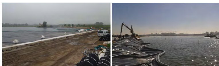
Figure 11: Deployment of Fabricated panels on North Dam
