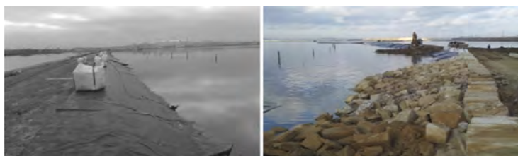
Figure 12: North Dam Geomembrane Installation
