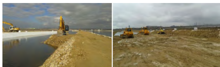
Figure 14: Road Dam Installation
