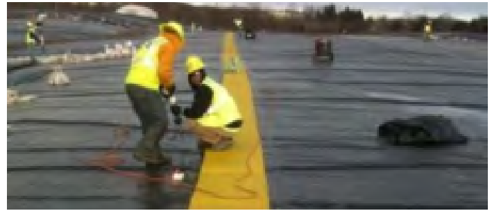
Installation of a slip resistant Walkmat on a geomembrane liner
