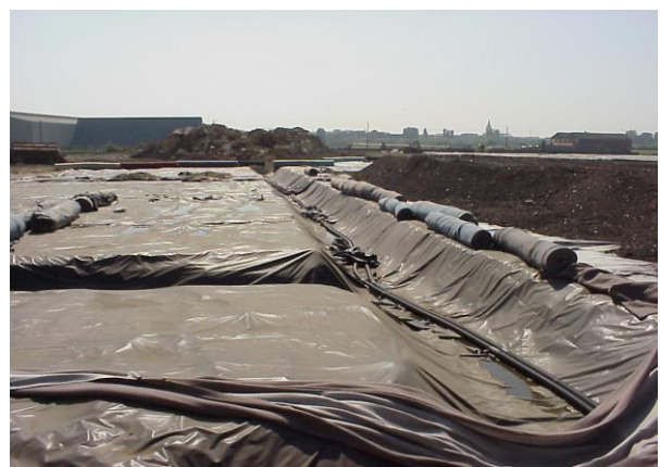
Figure 6. Geomembrane Cap Construction
