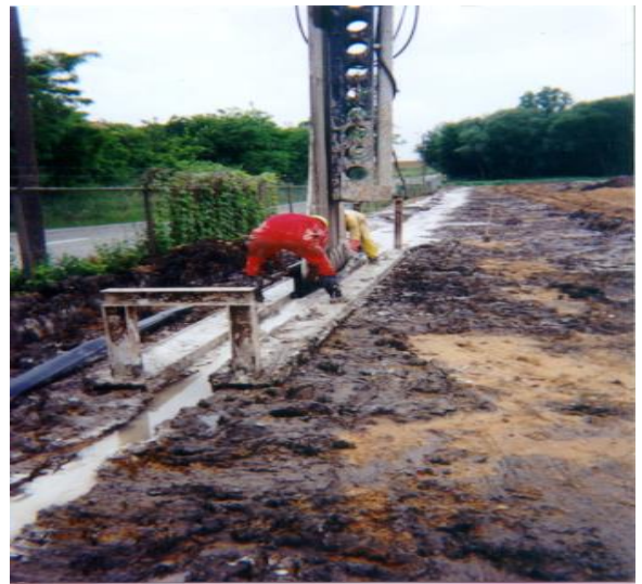
Figure 10. Geomembrane Wall Installation
