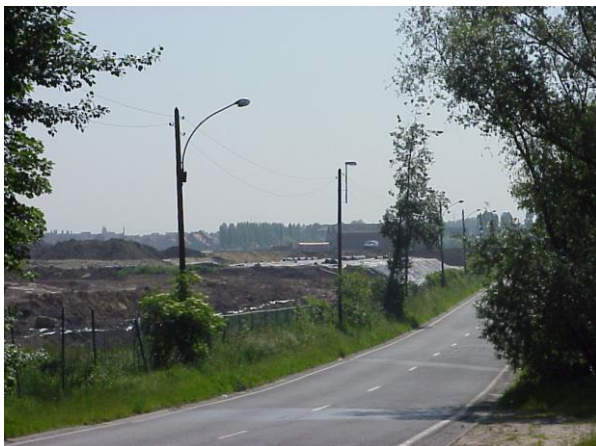
Figure 3. Site View from adjacent Road
