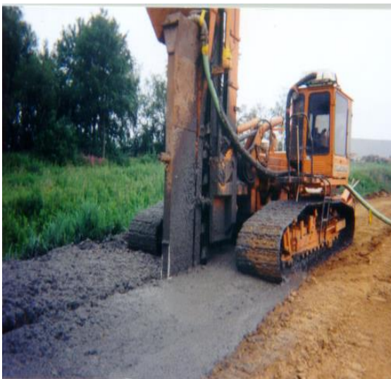
Figure 8. Bentonite-Cement Wall Installation
