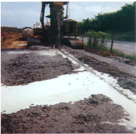
Figure 7. Bentonite –Cement Wall Installation
