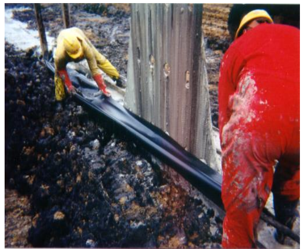
Figure 9. Geomembrane Wall Installation
