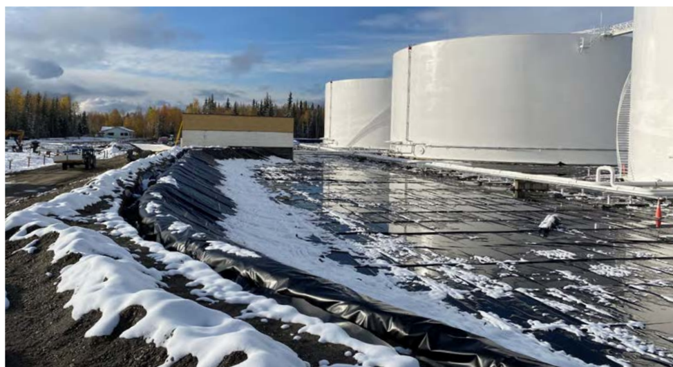
Figure 2 | XR-5 Ethylene Copolymer Geomembrane Lined Jet Fuel Secondary Containment Alaska, USA [photo source: Latitude 63]
