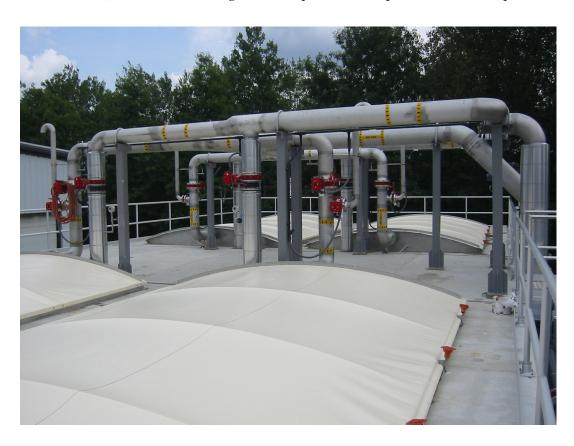
AnMBR system is a relatively new technology and was developed by ADI Systems, Inc. in Canada, in cooperation with Kubota Corporation of Japan. At Ken's Foods, the technology is used to process challenging wastewaters with high levels of organic content, while generating enough biogas to supply 100% of the heat required for the treatment plant's daily operation. The biogas is also sufficient for supplying hot water for other requirements at the plant.
