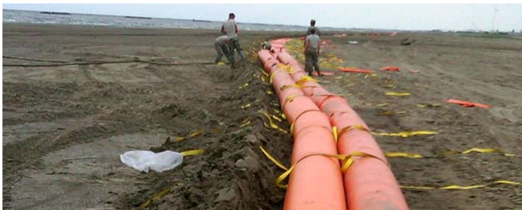
U.S. Flood Control installed 10 miles of Tiger Dams along the shores of Grand Isle beach in Louisiana, using Seaman Corporation's 28-ounce reinforced PVC geomembrane.
