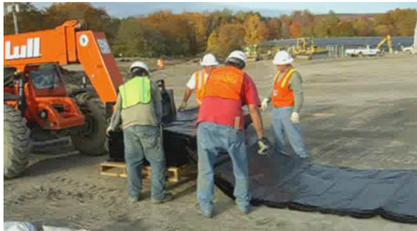
Prefabricated geomembrane panel being unfolded
