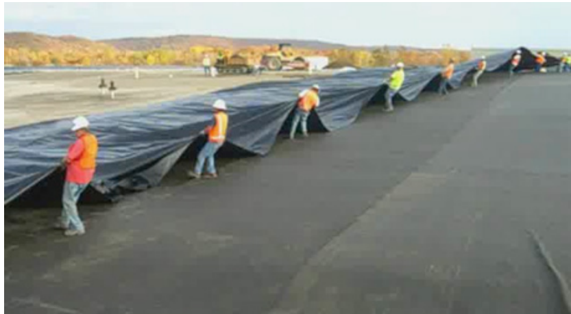
Prefabricated geomembrane panel (over 1/3 acre) being deployed over a geotextile fabric
