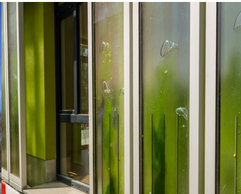
Photo 2: Close-up of the BIQ-Building façade
