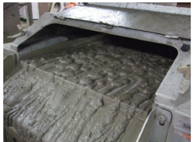
Fig. 5—Sand-slurry returns while dressing off at 1920 m RKB.
