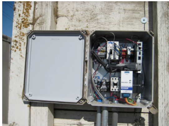
Figure 123: Polaris monitoring device and associated wiring.
