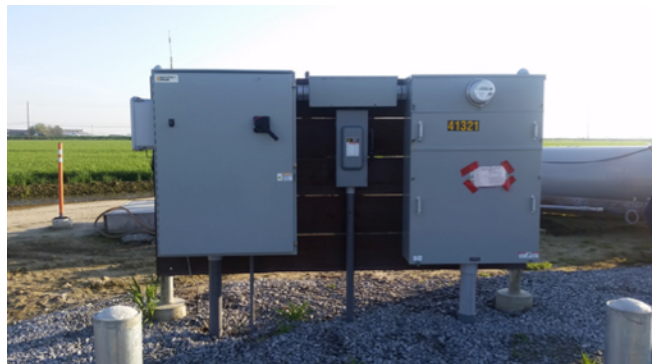
Figure 134: SCE meter, main service and motor electrical disconnect at the Dairy Well.
