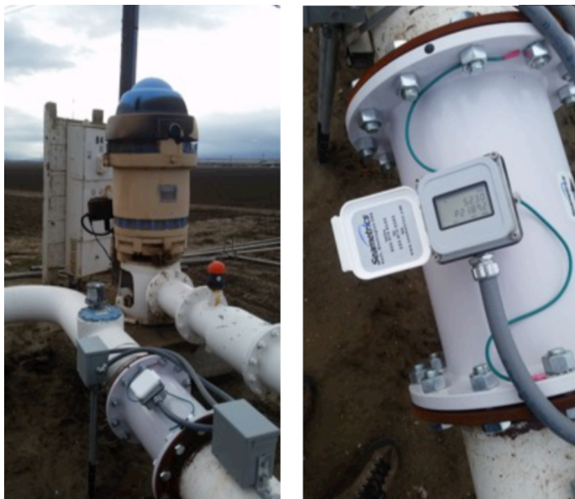
Figure 112: Flow meter interface and sectional view post installation.
