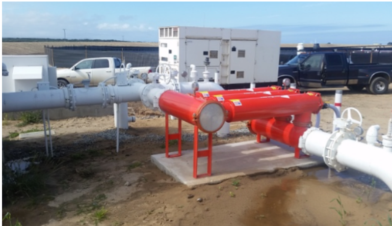
Figure 158: Sandhill Ranch reservoir pumps and filtration equipment.
