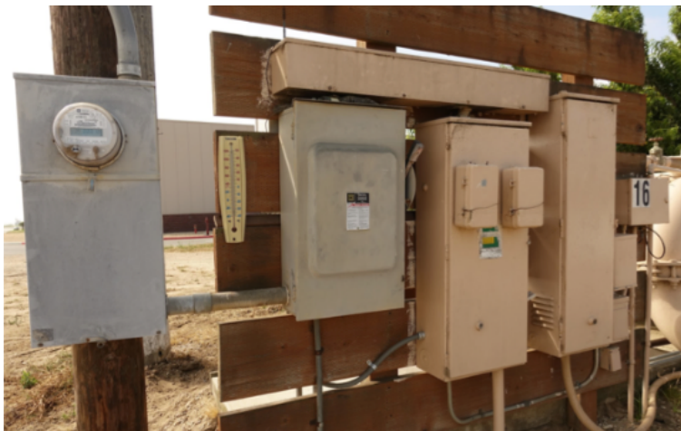
Figure 178: Utility meter and Polaris monitoring device
