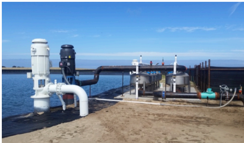
Figure 158: Sandhill Ranch reservoir pumps and filtration equipment.
