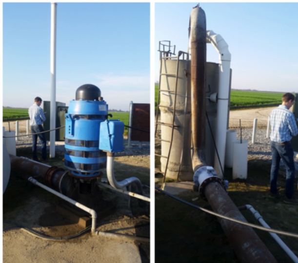
Figure 132: Irrigation pump and flow meter
