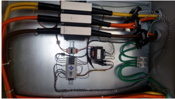
Figure 162: Sandhill Ranch energy monitoring meters.
