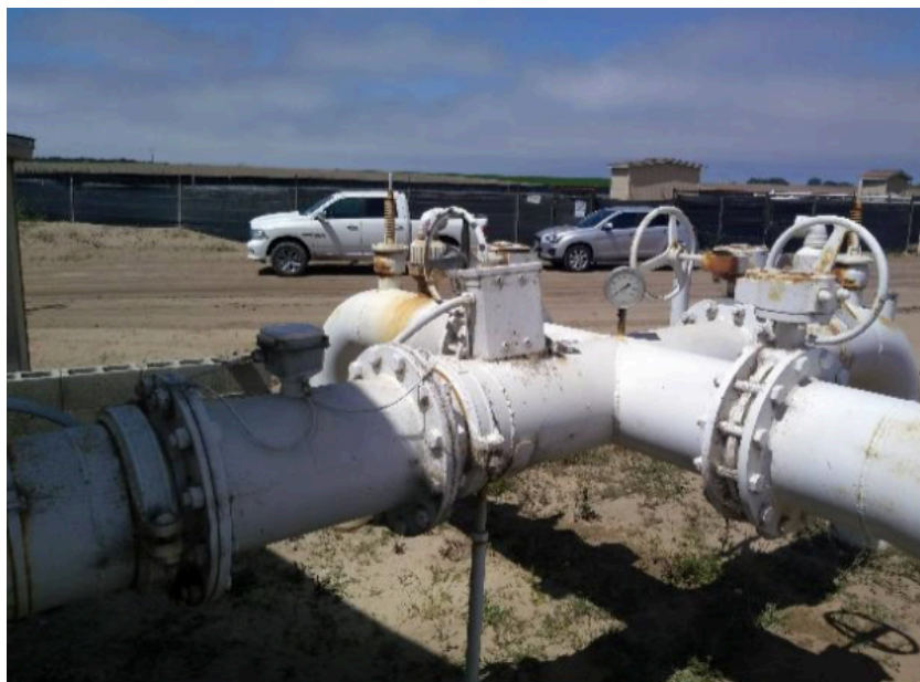
Figure 167: Sandhill ranch well reservoir flow Meter and Piping
