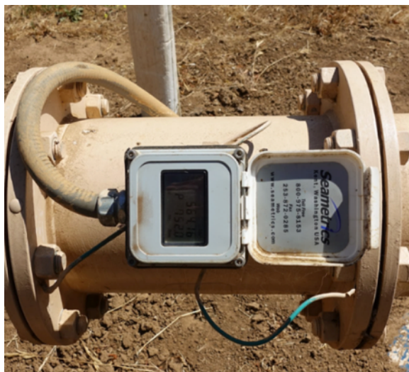
Figure 178: Utility meter and Polaris monitoring device
