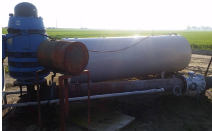
Figure 132: Irrigation pump and flow meter
