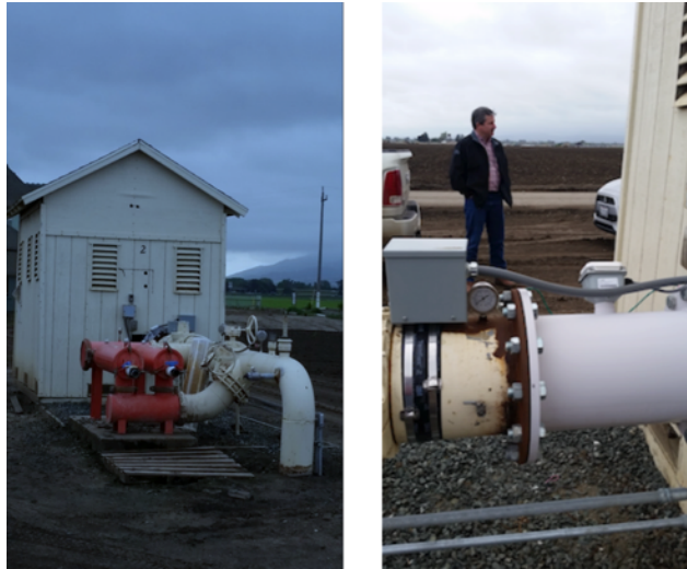
Figure 154: Pump flow meter at Davis Well #2
