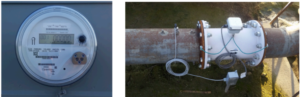
Figure 129: Newly installed Southern California Edison (SCE) electric utility meter and recently installed section of pipe, flow meter, pressure sensor, and associated wiring.
