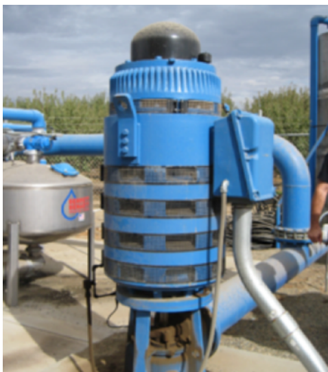
Figure 138: Goshen Ranch close up of Well pump motor
