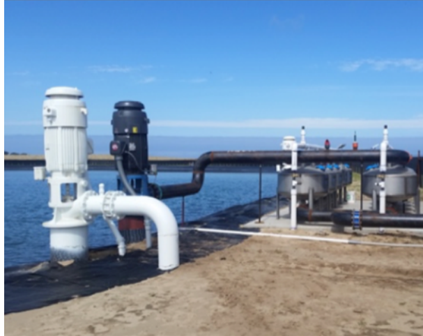
Figure 69: Ranch reservoir pumps & filtration equipment
