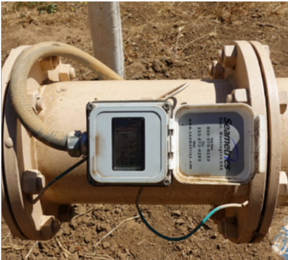
Figure 88: Newly installed digital flow meter at an irrigation pump
