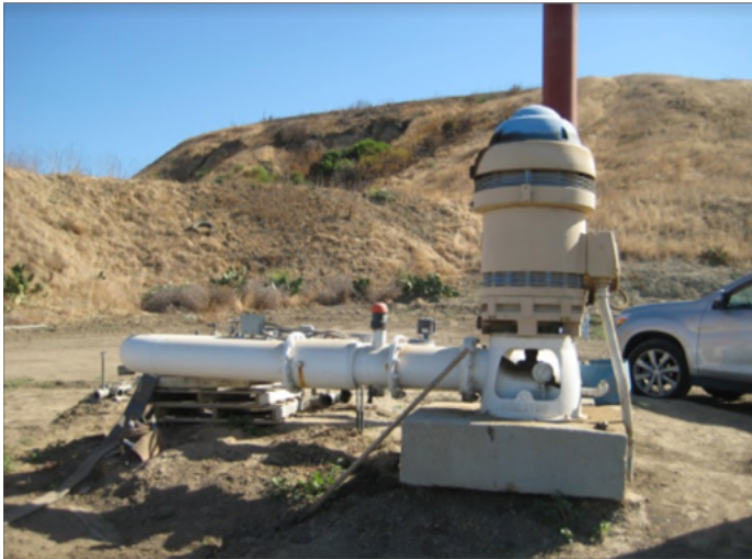
Figure 30: PG&E electric meter, installed digital flow meter, pump motor & well
