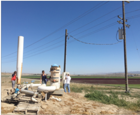
Figure 19: Project team members surveying an irrigation pump tied to a PG&E utility pole/transformer & electric meter with old analog flow meter
