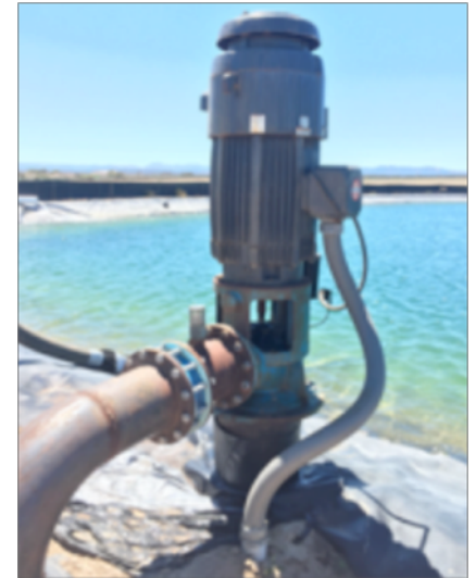
Figure 61: Booster pump and reservoir
