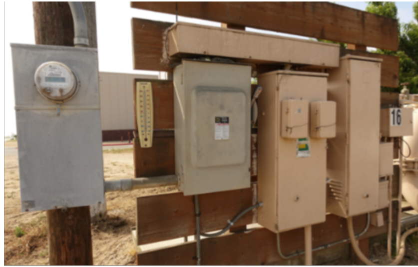
Figure 89: PG&E utility meter & switchgear with newly installed Polaris monitoring hardware
