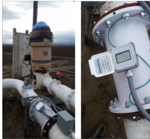
Figure 23: Newly installed digital flow meter & pipe section at an irrigation pump
