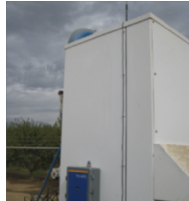
Figure 47: Polaris device & antenna installed at ranch well with variable frequency drive (VFD) enclosure
