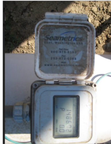
Figure 33: Installed digital flow meter
