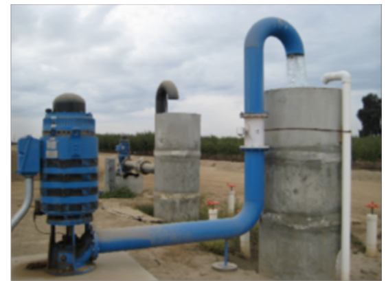
Figure 54: Almond ranch well pump in operation
