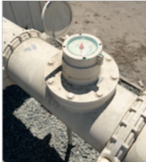
Figure 59: Surveying an irrigation well pump house & old analog flow meter with berry grower staff
