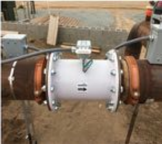
Figure 62: Installed digital flow meter & pressure sensor
