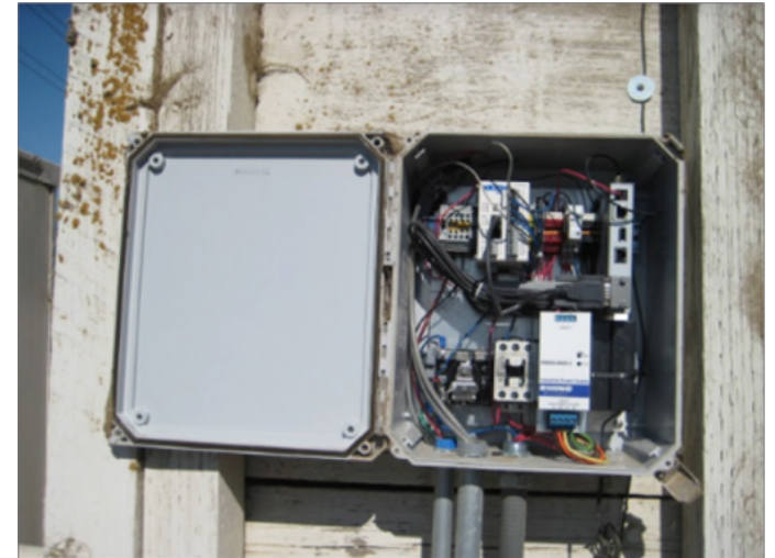
Figure 34: Installed Polaris monitoring device & associated wiring
