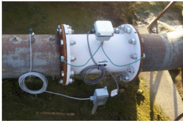
Figure 40: Newly installed SCE electric utility meter, pipe section, flow meter, pressure sensor & associated wiring
