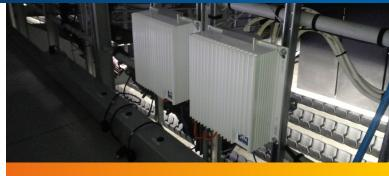
Two remote units are deployed on the catwalk to help ensure **powerful cellular coverage is available throughout the arena.**
