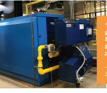
Last fall, GTW was selected by Marie to replace critical boilers in two buildings. We installed two Buderus hydronic cast iron boilers, each with a Power Flame burner and Mini 8 AutoFlame controls.
