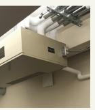
The Wilkinson team removed the two old steam boilers and put in a hydronic system. This involved the installation of a 4 pipe heating and AC system for the classrooms in the upper and lower schools.
