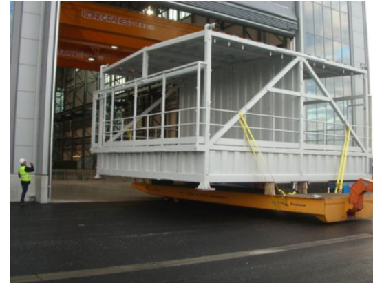
Skidding upper module into workshop
