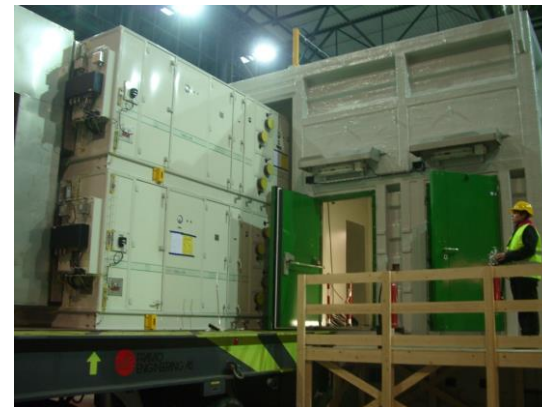
Installation of HVAC Units
