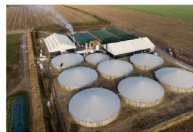
External silos of the farm in Skive, Denmark.
