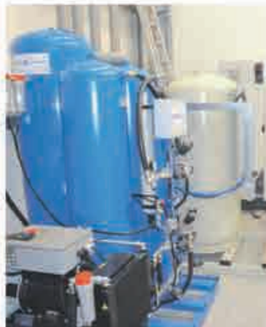
On the right (in blue colour) airo generators; on the left (in grey colour) CO 2 adsorbents; both of them contribute to generation of high quality controlled atmosphere. Controlled atmosphere allows for lengthening the shelf-life of foods by slowing down and postpone the ripening. To maintain high standards the Besseling Group has chosen Mattei compressors.
