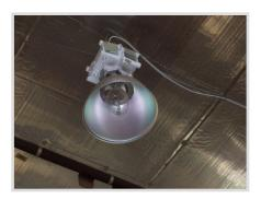
Most existing High Bay Lighting and Low Bay Lighting applications utilize High Intensity Discharge (HID) lamps such as Metal Halide, High Pressure Sodium, and if they are very hold, Mercury Vapor Lamps.
