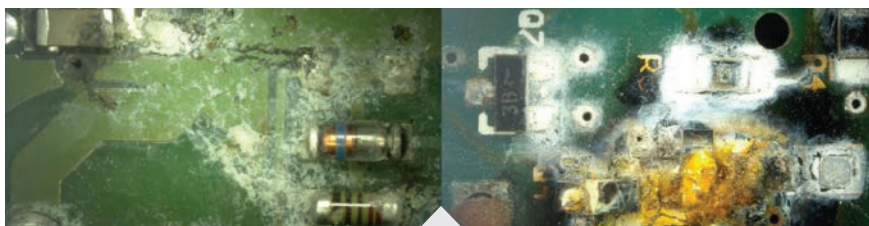
Image 7: Damage caused by electrochemical migration (left) and dielectric breakdown (right)
