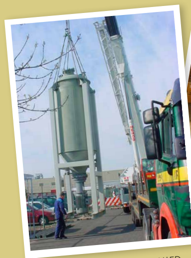
CONTACTOR BEING INSTALLED IN HEIJNINGEN (NL)
