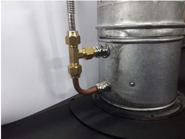
Figure 24: Pressure Switch Connection to the Chimney
