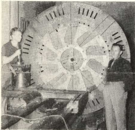
TYPICAL WEAR PLATE from an 84-inch chipper disc following application of Colmonoy No. 5.
