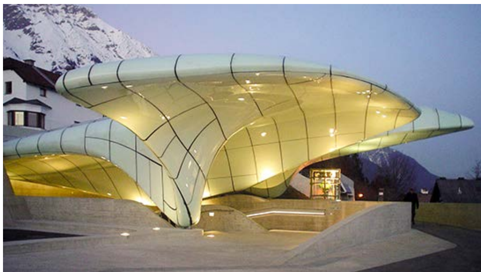
Zaha Hadid's Nordpark Railway Stations used heat-bending techniques to achieve double curvatures.
