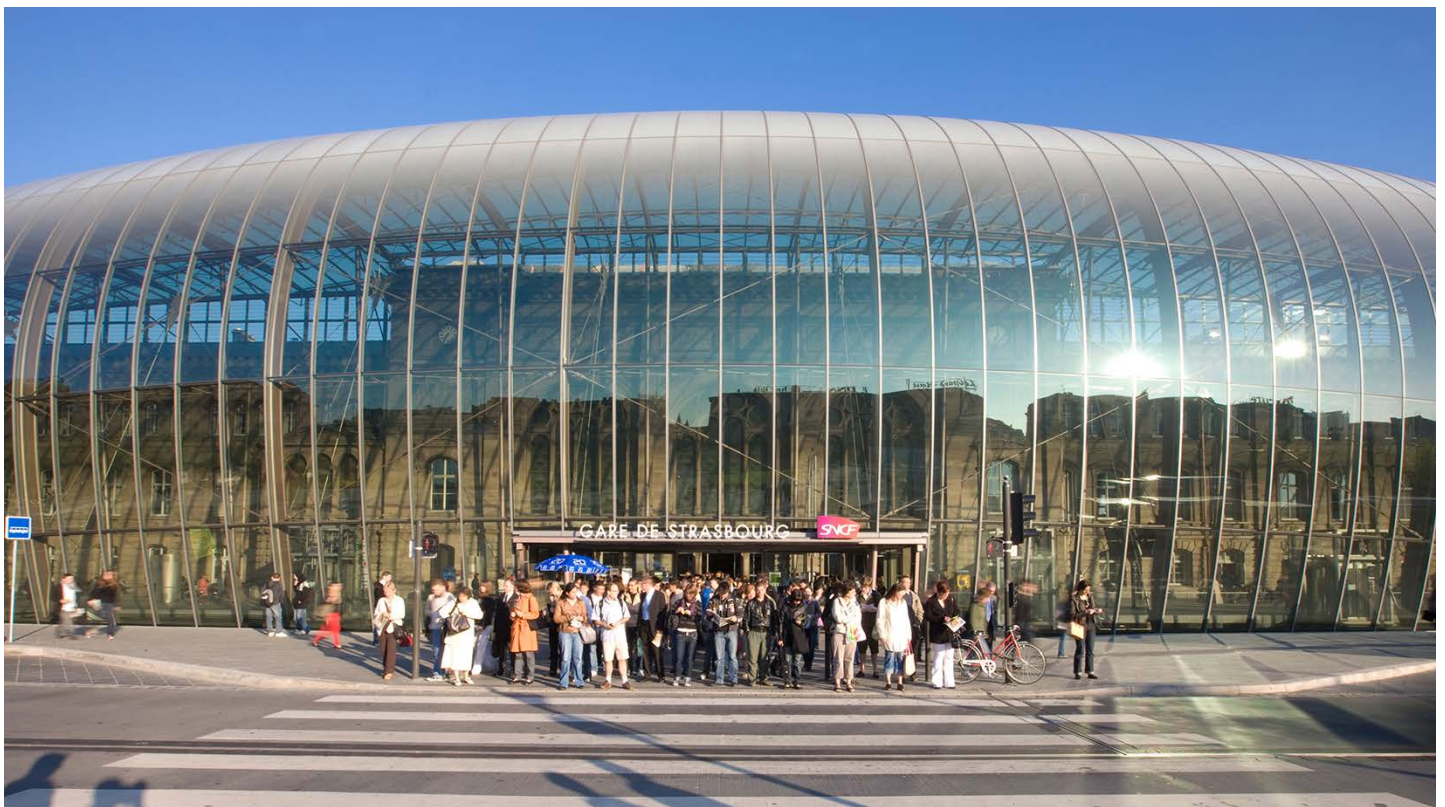
The Gare de Strasbourg in Bas-Rhin, France utilized a cold bending technique called lamination bending to achieve its flat and uniform appearance, while also reducing energy and cost. Photo courtesy of Sedak.
