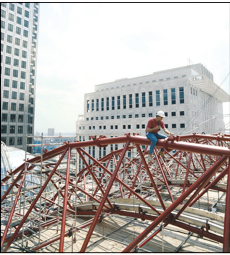
Weissbach, 1990, inspecting a skylight over the railway at Canary Wharf, London, England.
