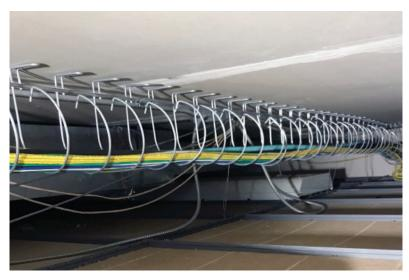
runs. Available in three loading diameters of 2", 4" and 6", the 454 Series can reliably hold bundles of up to 30, 120, or 260 Category 6 cables (.25 in²) respectively. Designed for easy cable pulling or loading from the side, 454 Series cable tray sections are joined together using universal inline connector bolts that provide both mechanical and electrical bonding in one piece.
