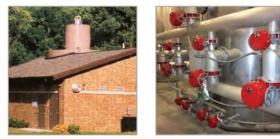
AERALATER package plants can be designed for outdoor or partial indoor installation. Units can be designed with the aeration or detention section penetrating the building roof. This helps save building size and cost.
