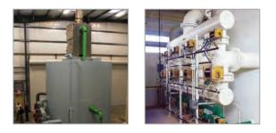
All AERALATER units are provided with a control cabinet for operation of the well pumps and high-service pumps based on the water level in the storage tank. The panel also operates the aerator blower and chemical feeders, based on the operation of the well pumps. When desired, control systems are provided to automatically step the AERALATER through a backwash and return it to service.
