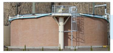
WesTech ExtremeDuty Sludge Mixers provide vigorous mixing of digester contents to prevent stratification and improve the anaerobic process.
