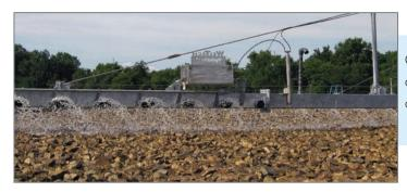
Controlling the dosing rate of the trickling filter is the key feature of the HydroDoc. WesTech has successfully provided hundreds of distributors that offer these process advantages.
