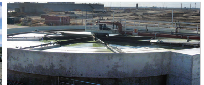
Rectangular tanks are easier to install while circular DAF designs require less maintenance
