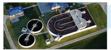
The OxyStream<sup>™</sup> oxidation ditch system combines slow-speed surface aerators with an oxidation ditch design based on site-specific conditions and WesTech's proprietary hydraulic model.
