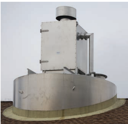
The flexible membrane provides a very effective seal with the roof.
