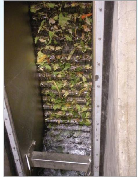
**Efficient screenings capture protects the downstream sand filters**
