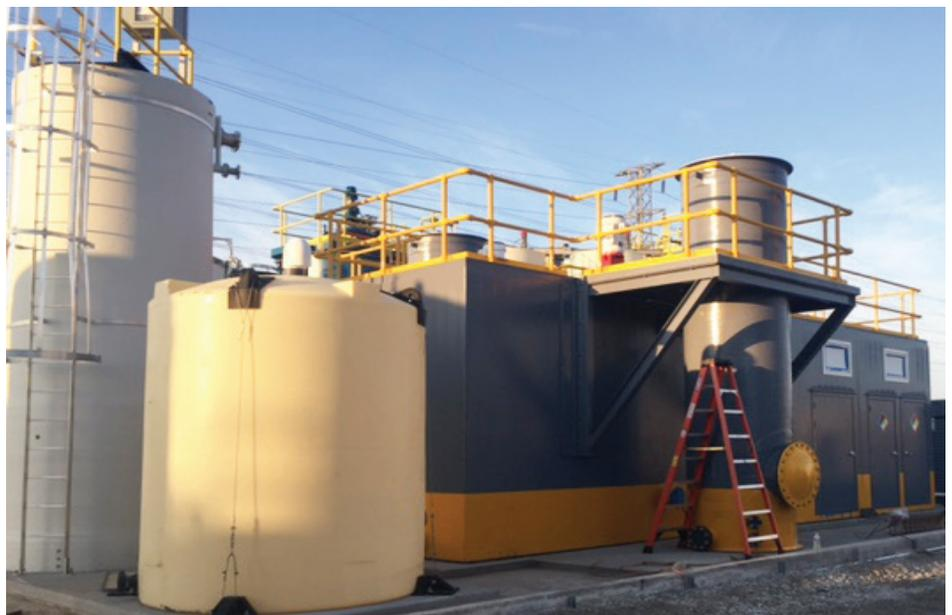
The water was then fed into the second half of the treatment train, which consisted of a sand filter followed by a biological treatment system for selenium reduction.
