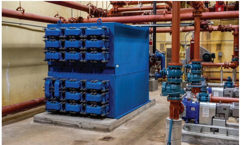
Tube-in-tube heat exchanger
