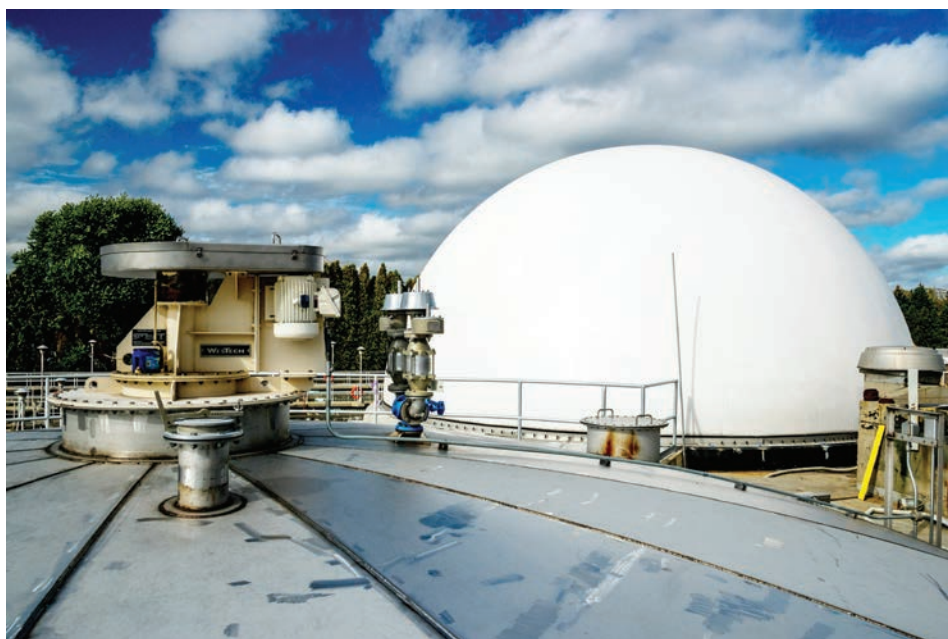
New stainless steel cover and DuoSphere dual membrane gas holder
