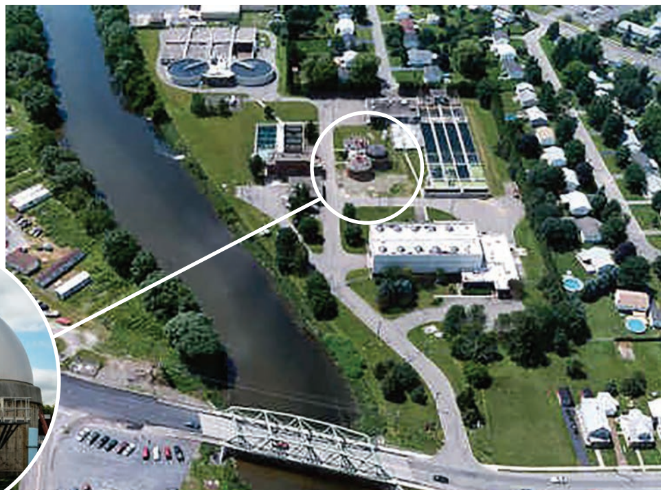
Before: The Cortland Wastewater Treatment Plant with anaerobic digestion site indicated by the circle
