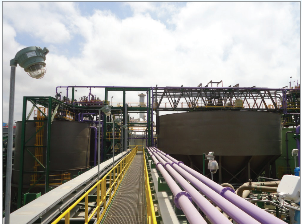
WesTech 20m Deep Bed™ paste thickener and 10m surge tanks feeding the acid plant.
