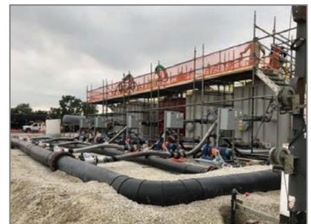
The mobile clarifier unit can handle a total suspended solids (TSS) load of up to 6,000 mg/L with integral sludge pumps that are already piped, wired, and ready for service.
