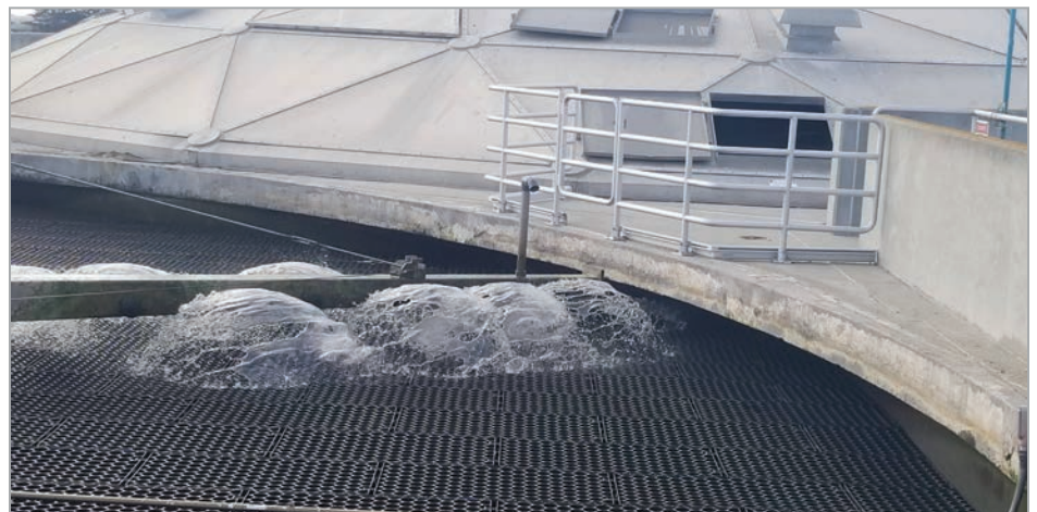
Testing of Nozzle Under Deck
