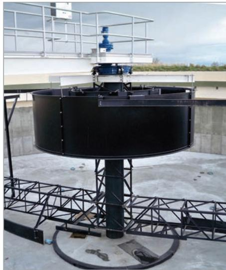
**COP: Rapid Sludge Removal Components**
