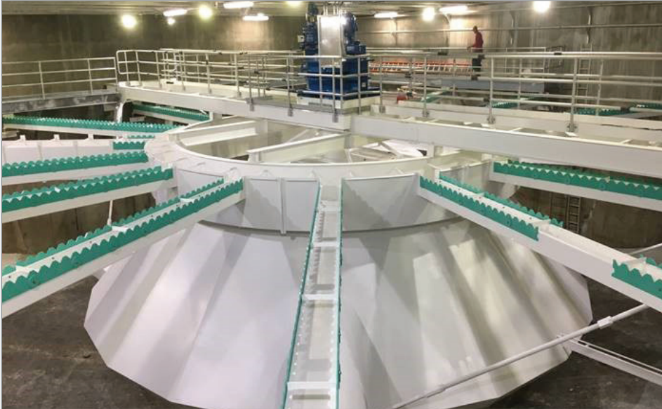
Solids CONTACT CLARIFIER Under Construction
