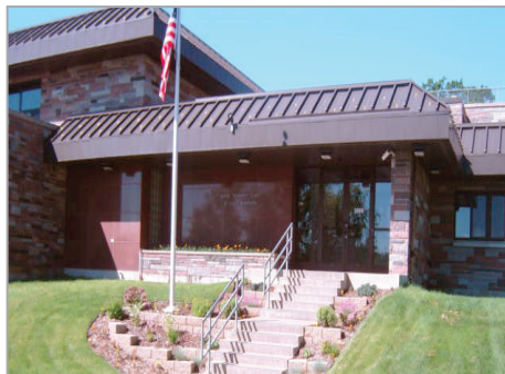
The St. Cloud Water Treatment Facility's Main Entrance
