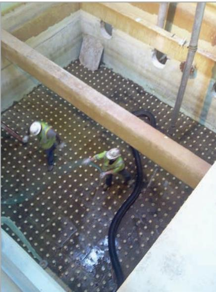
Webster City moved forward with installing the WesTech MULTIWASH backwash enhancement. The plant's filter runs are now in excess of 100 hours. MULTIWASH also provides a vigorous backwash which efficiently cleans the filter media, eliminating the plant's concern that a water-only backwash would not adequately clean the media. MULTIWASH troughs have low-profile media retaining baffles to help with the plant's media retention.
