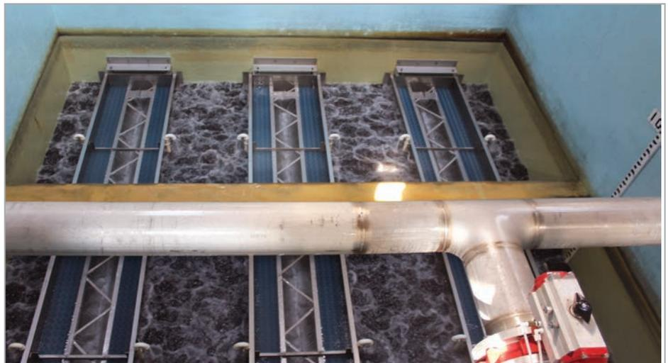
Another challenge to installing the washtroughs into the filter cells was working around a concrete beam located in the middle of the cells. The solution was to modify the original washtrough design so the contractor could angle the troughs around the concrete beam.
