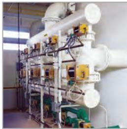
All AERALATER units are provided with a control cabinet for operation of the well pumps and high-service pumps based on the water level in the storage tank. The panel also operates the aerator blower and chemical feeders, based on the operation of the well pumps. When desired, control systems are provided to automatically step the AERALATER through a backwash and return it to service.
