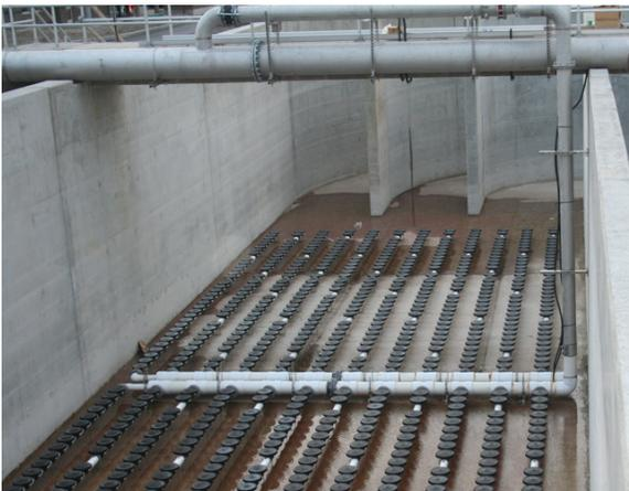
Fine bubble diffusers installed on the bottom of the channel provide the aeration. When other types of mixers are used, the local diffuser density (quantity per sq. ft.) may need to be higher due to both the position of the mixer and the required mixer clearance. An elevated diffuser density leads to decreased oxygen transfer efficiency, a problem solved with the Landox.
