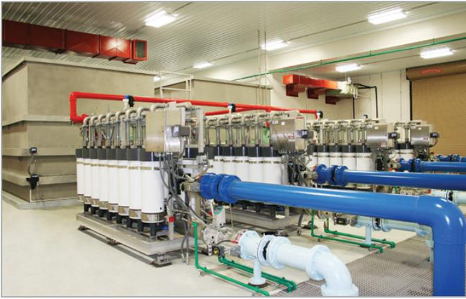
The **AltaFilter™ Ultrafiltration System** is supplied as a pre-engineered system with integrated piping, valves and controls, and has been successfully applied in potable water treatment, municipal wastewater filtration and industrial applications. Custom-engineered systems are available to meet unique needs.
