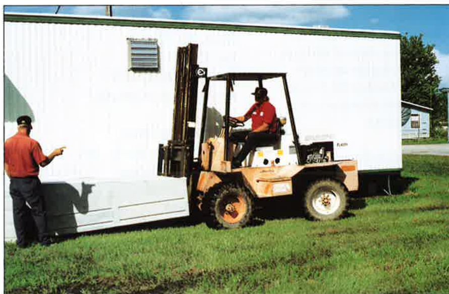
Lightweight components are manufactured with 2" steel reinforced side walls. This feature eliminates hazardous open crawl spaces while adding stability and strength.
