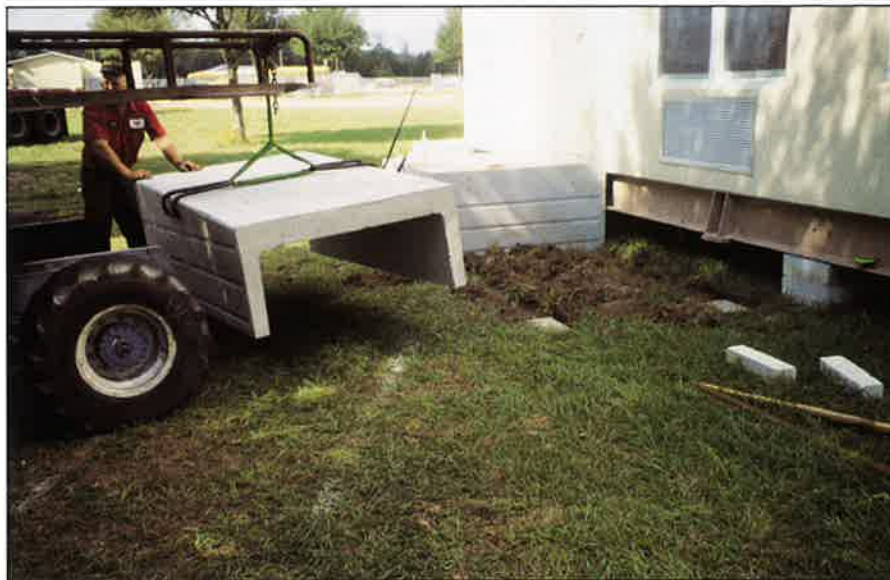
Modular Ramp and Step Units have skirts on three sides and are easily installed and relocated
