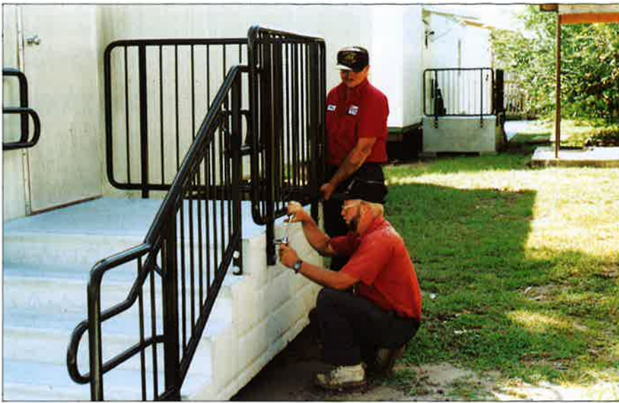
Railings and anchor bolts are provided and can be installed in minutes using hand tools.
