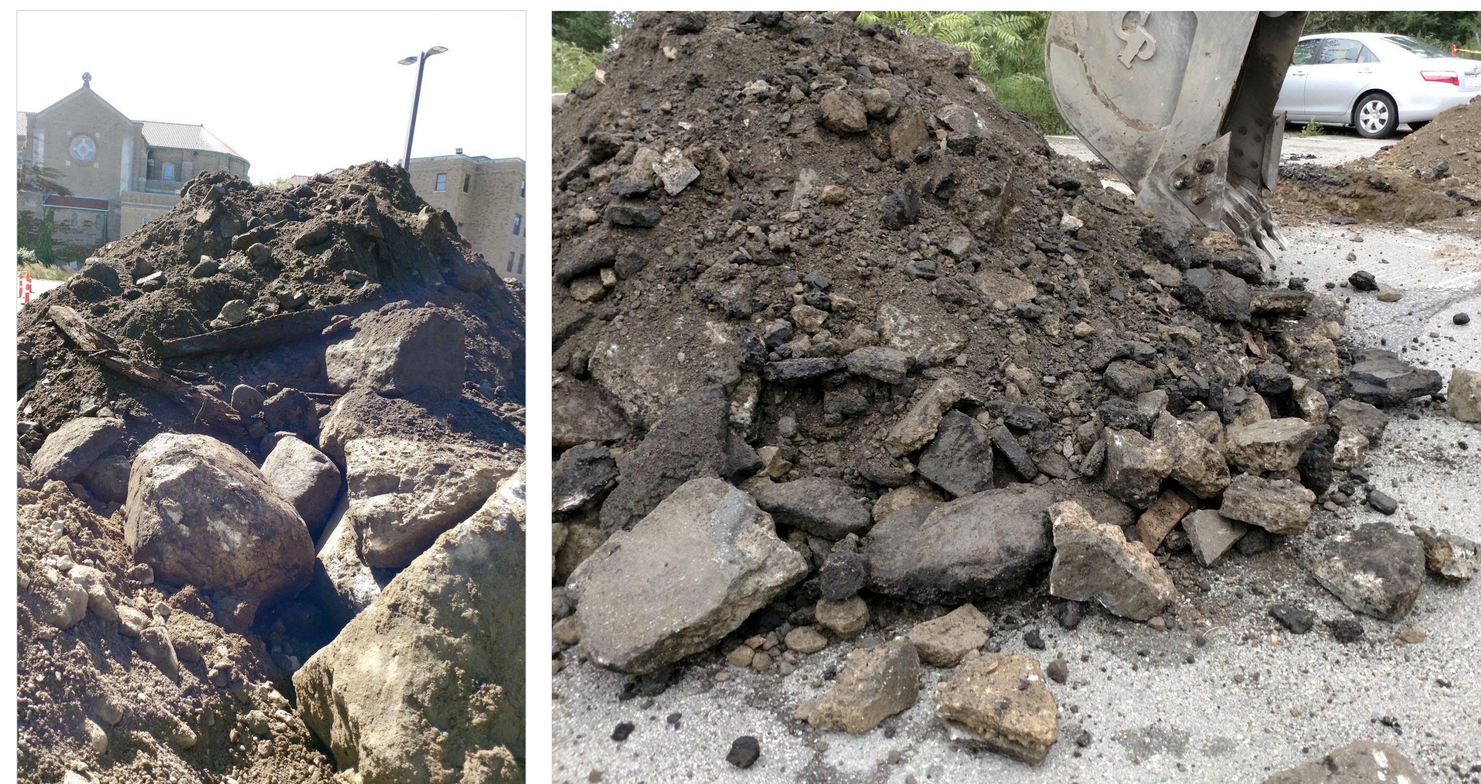
Examples of debris in the fill
